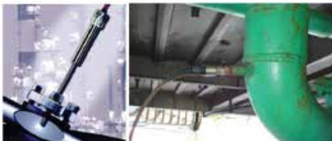
levels to ensure the discharge is within the local environmental regulatory compliance limits. For all Model 6650SP installations, and for particularly remote sensing applications such as this, TAI provides the fiber optic cables in a flexible conduit to protect the fibers from being accidentally mishandled.
