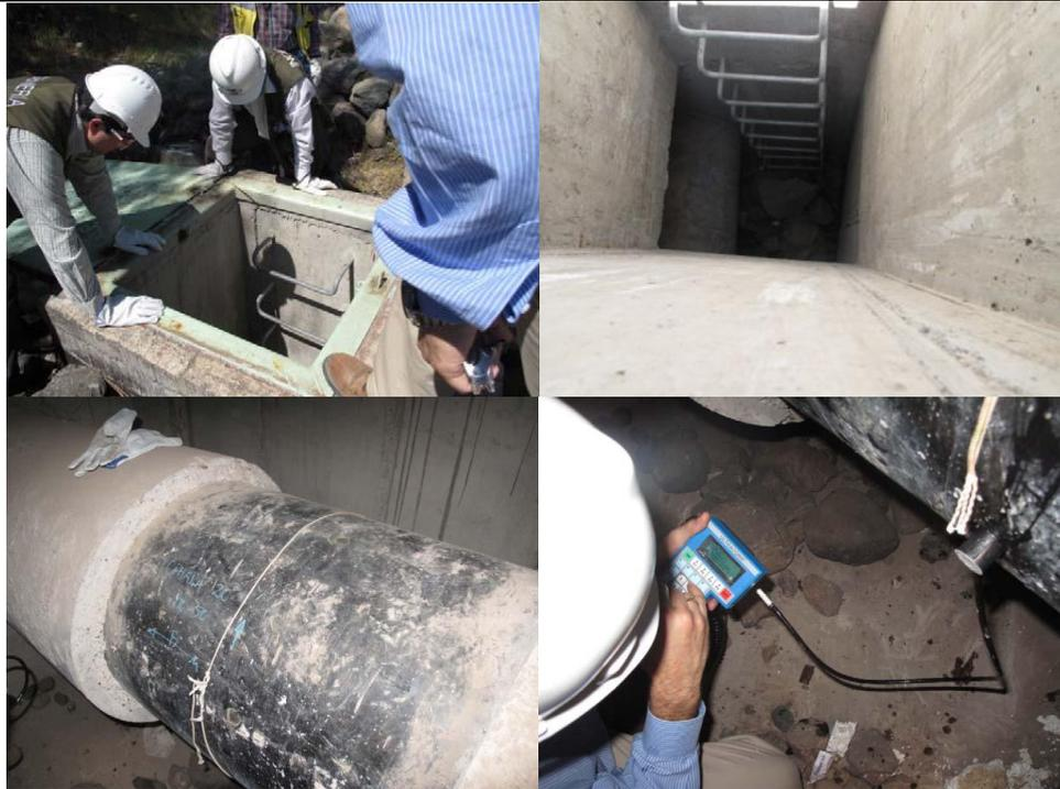
Figure 3 - buried enclosure for an existent pipeline
